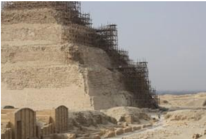
Scaffolding covers large portions of the pyramid side
